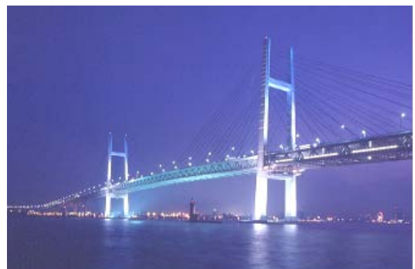
▲Yokohama Bay Bridge
