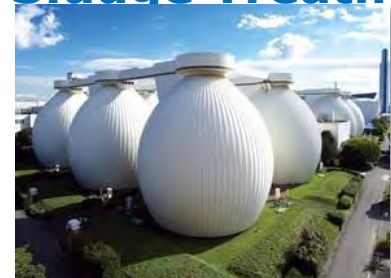
Sludge Biogas Plant
