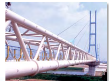
Water Pipe Bridge
