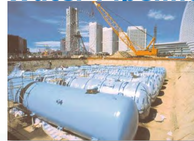
Anti-Seismic Tank (Yokohama)
