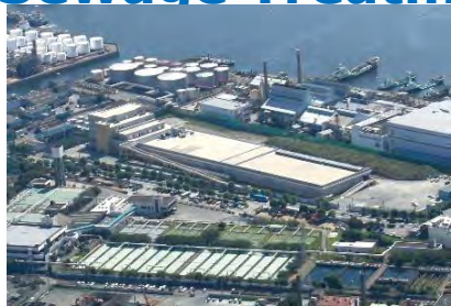
Iriezaki Sewage Treatment Plant
