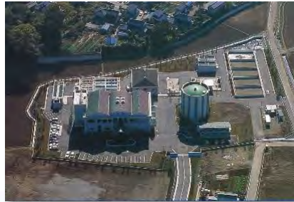
Kawazuma Water Treatment Plant
