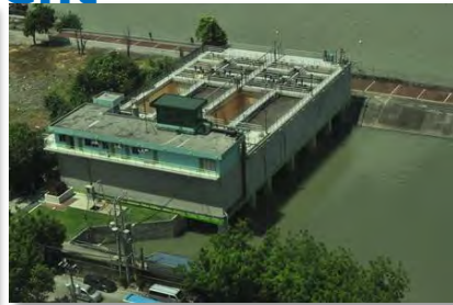
Sewage Treatment Plant (Philippines)
